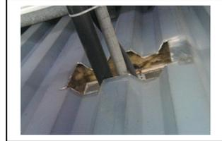
A fire will spread easily and quickly through holes and gaps like these left by workmen and builders. Such oversight is very common indeed. **A fire will spread through a hole the size of a pencil in four minutes.**
