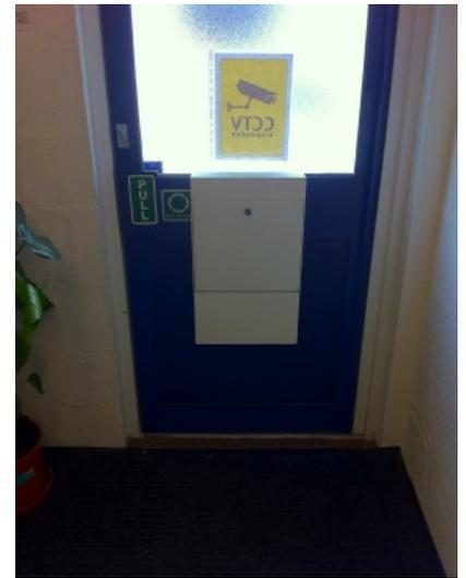
Image of letterbox mounted onto door over letterbox; and showing extinguisher strip around inside
